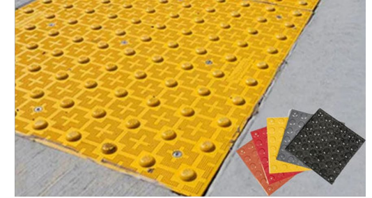
Detectable warning surface example – S03, S06, S08-S10
