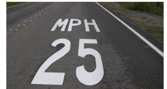
Speed limit pavement marking example from FHWA - S14
