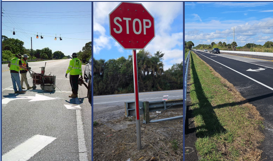
Road striping and markings replaced Reflective strips added to Stop sign Right-turn lane added
