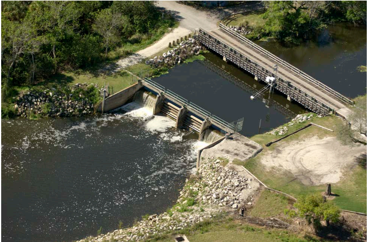
Water control structure on Ten Mile Creek at Gordy Road in St. Lucie County. Photo courtesy of SFWMD.
