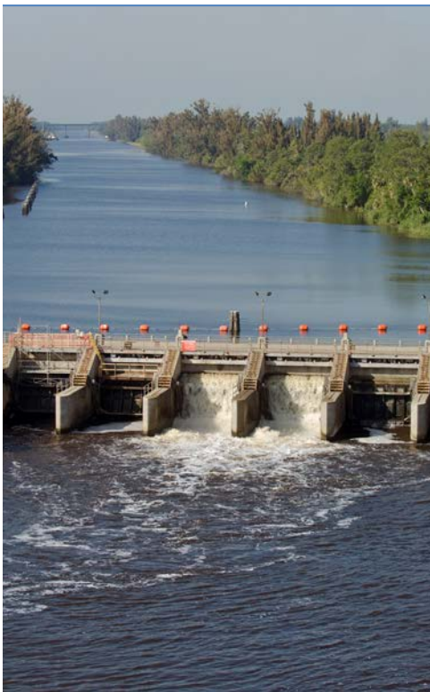
S-80 structure. Photo courtesy of SFWMD
