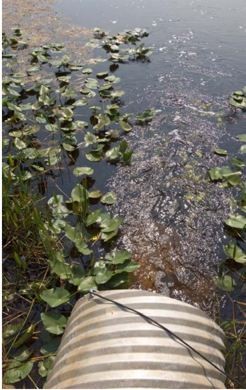
Outfall. Photo courtesy of SFWMD
