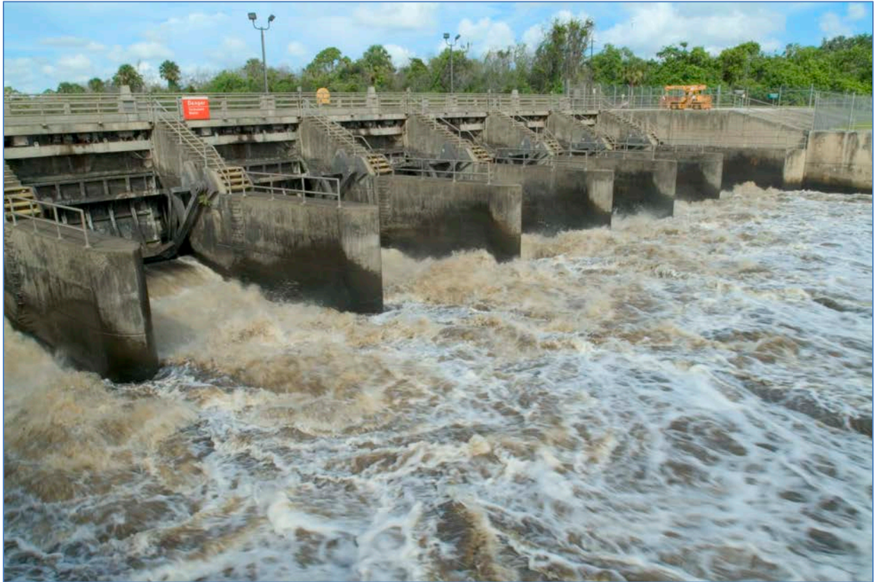
Discharges from Lake Okeechobee flow through the S-80 structure on the C-44 canal. Photo courtesy of SFWMD.
