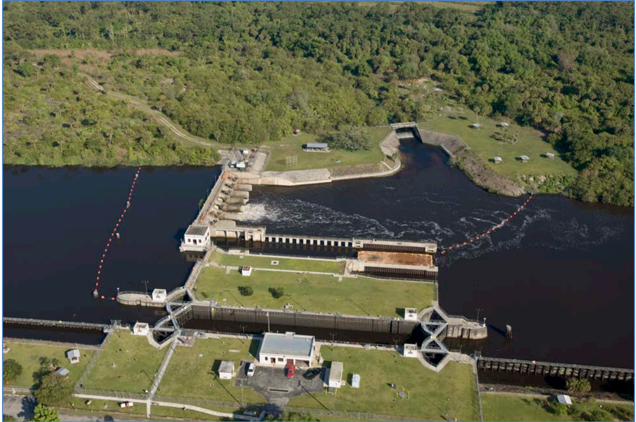
S-80 structure and the St. Lucie Lock on the C-44 canal. Photo courtesy of SFWMD.
