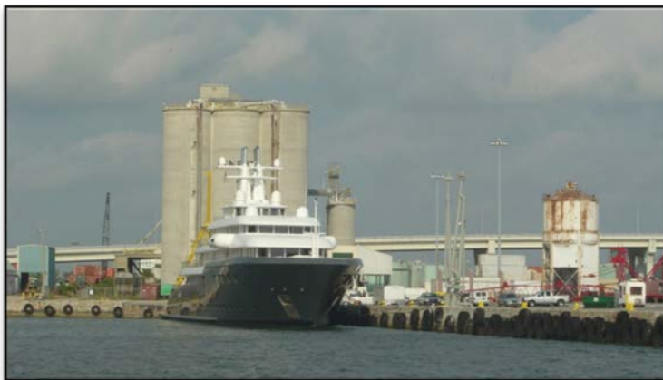
The Port of Fort Pierce Master Plan considers the continued handling of niche cargo, and it was recently listed as an “emerging port” by the State of Florida.
