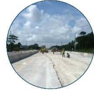
New Roads/Widen Roads and Bridges
