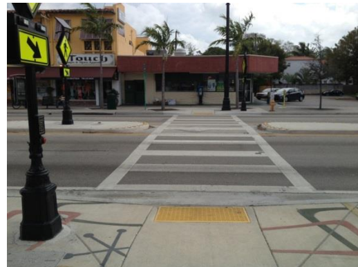
Rectangular rapid flashing beacon (RRFB) mid-block crosswalk on a five-lane arterial roadway
