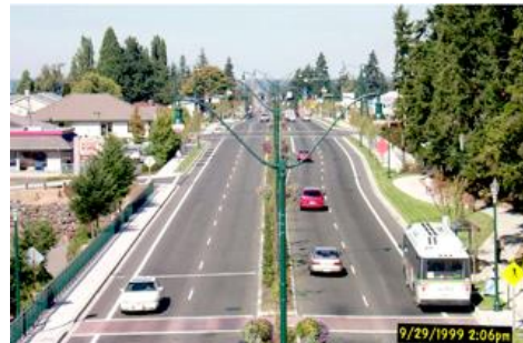
Bridgeport Way after transformation: University Place, WA
