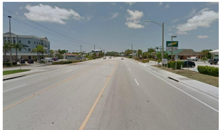
East Ocean Boulevard with center two-way left-turn lane, east of SE Monterey Road, looking west
