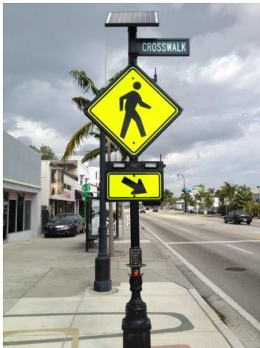
Rectangular rapid flashing beacon (RRFB) device on a five-lane arterial roadway
