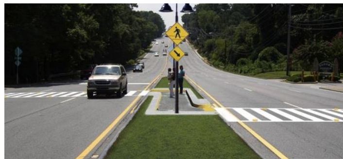
Staggered pedestrian crossing with raised concrete island median refuge
