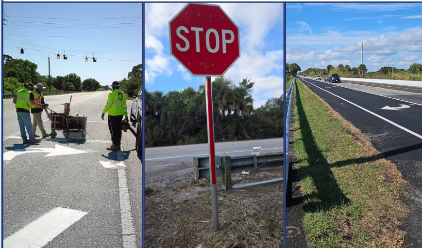
Road striping and markings replaced Reflective strips added to Stop sign Right-turn lane added MPO Policy Board 9/21/26
