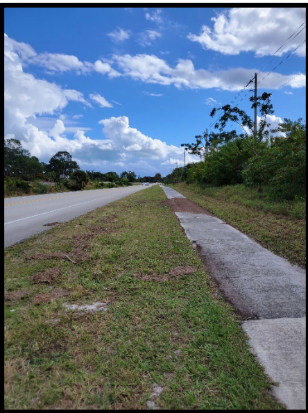
Figure 28: Evidence of Sidewalk Flooding
