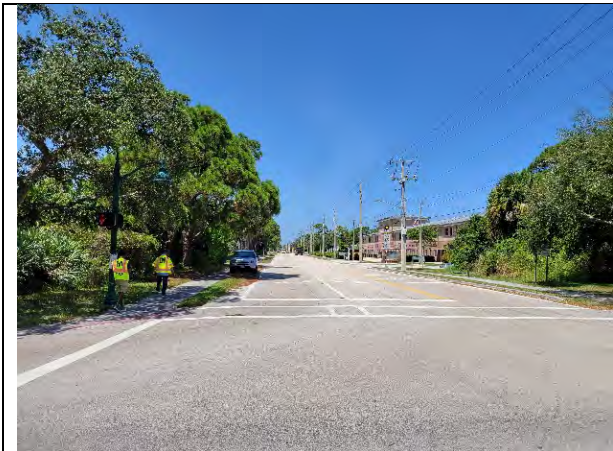
Gomez Avenue at Bridge Road – Sidewalks on Both Sides - North
