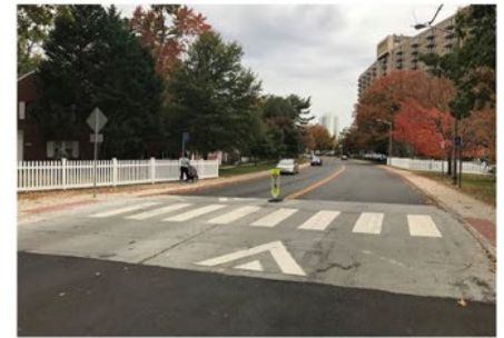
Raised Pedestrian Crossing
