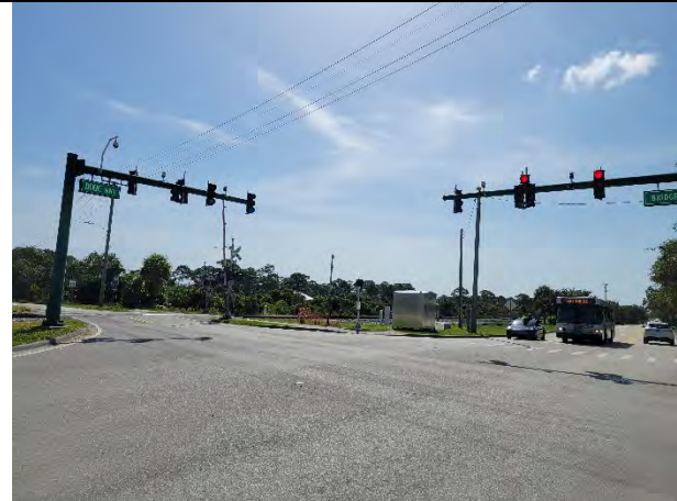
Dixie Highway & Bridge Road Intersection – NWC
