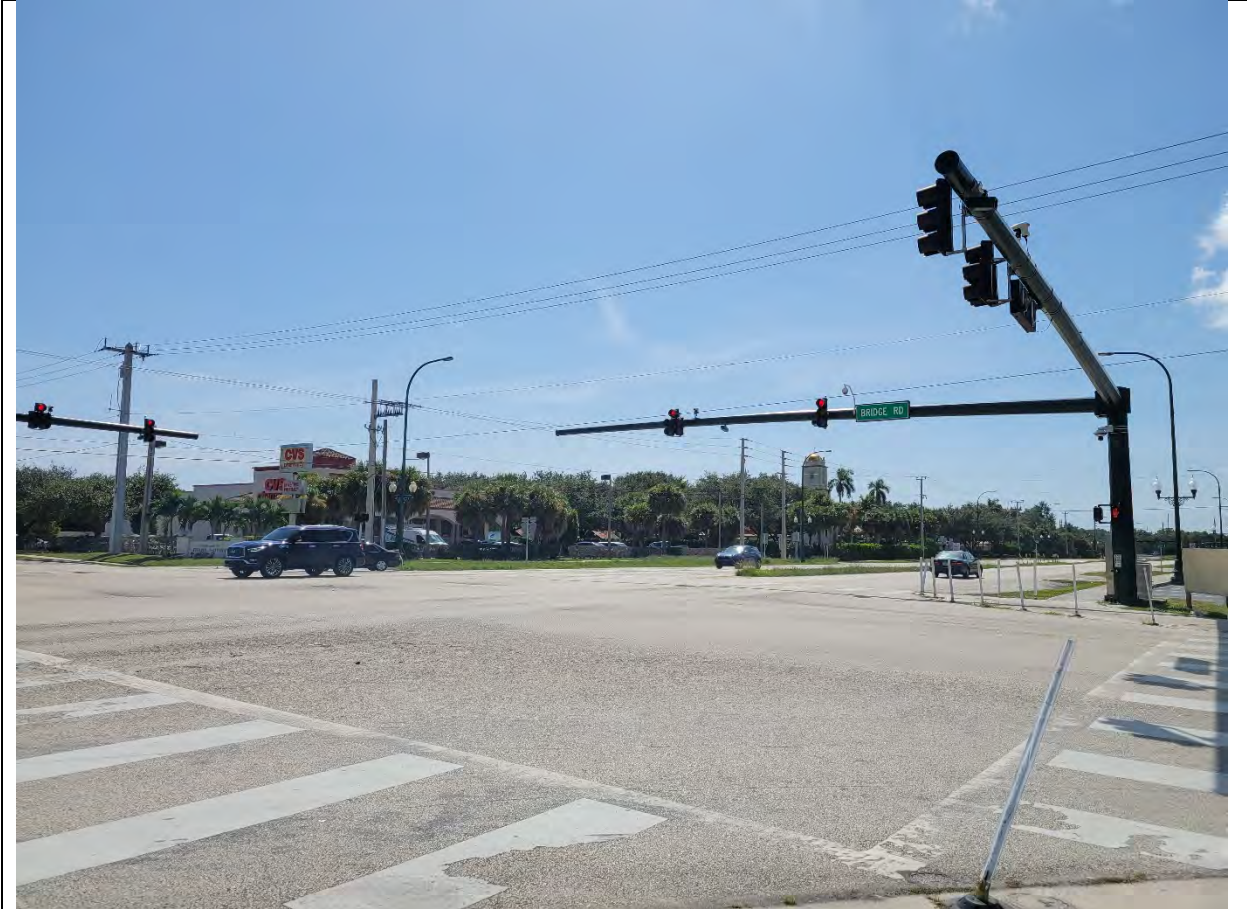
Intersection at US 1 & Bridge Rd (NWC) - Southeast
