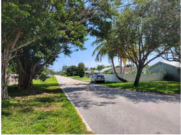
Sidewalk Missing on South Side of Crossrip Street - East
