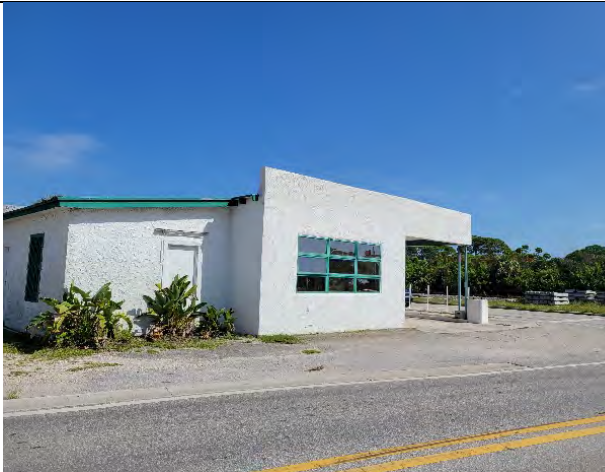
Missing Sidewalk Near Dixie Hwy - Northeast
