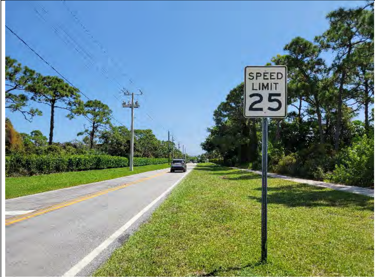
Sidewalks on South Side, No Sidewalk on North Side of Osprey Street - East
