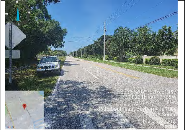
Sidewalks Missing on East Side of Gomez Ave - North
