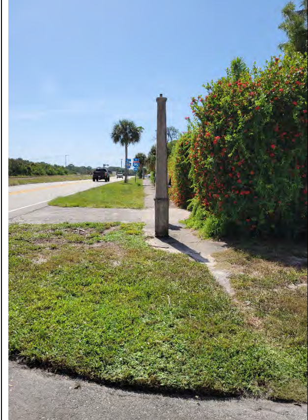
Ped Path/Missing Sidewalk Segment, Light Pole Obstructing Sidewalk (77.5") near Wittman Textiles - South
