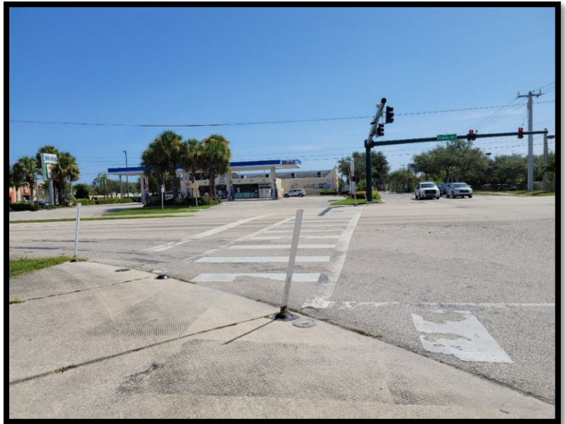
Figure 30: Intersection of SR-5 & Bridge Rd looking east from the northwest corner
