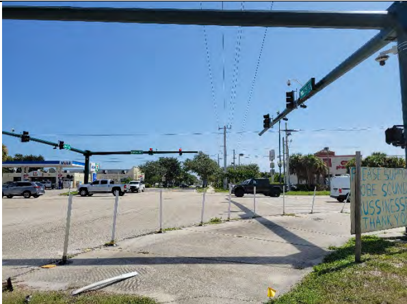
SWC Protected by Multiple Delineators, Missing Tactile Surface - East
