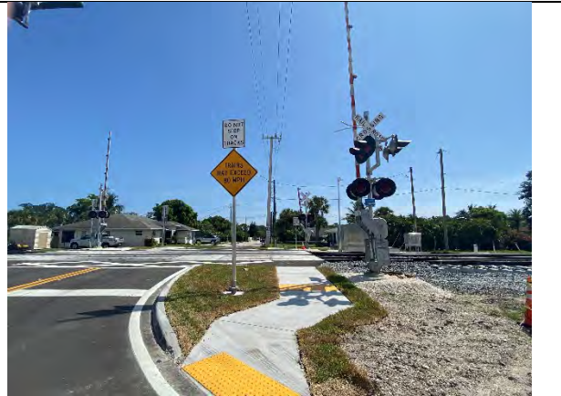
Pettway Street Sidewalks on both sides - East
