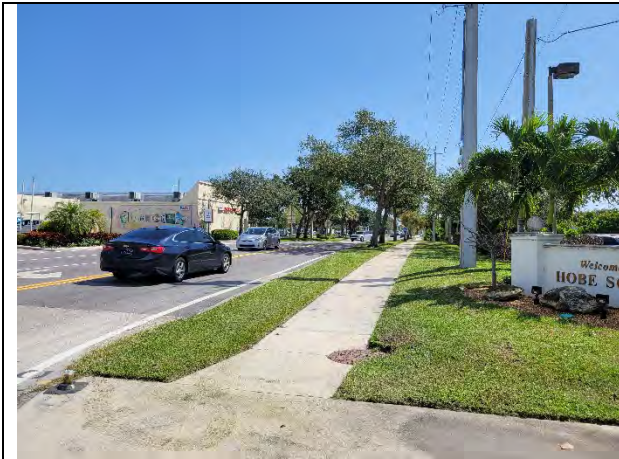
South Side Sidewalk, Missing North Side – At US 1 - East
