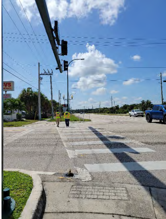
East Leg Crosswalk (NEC) – Missing Delineators and Tactile Surface - South
