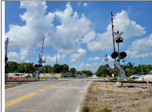
Crossrip Street near Dixie Highway, Sidewalks Missing over Railroad Crossing – West
