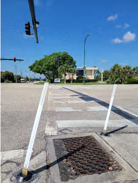
North Leg Crosswalk (NEC) – Drainage Grate, Faded Crosswalks, Delineators Partially Obstructing Pathway, Missing Tactile Surface - West
