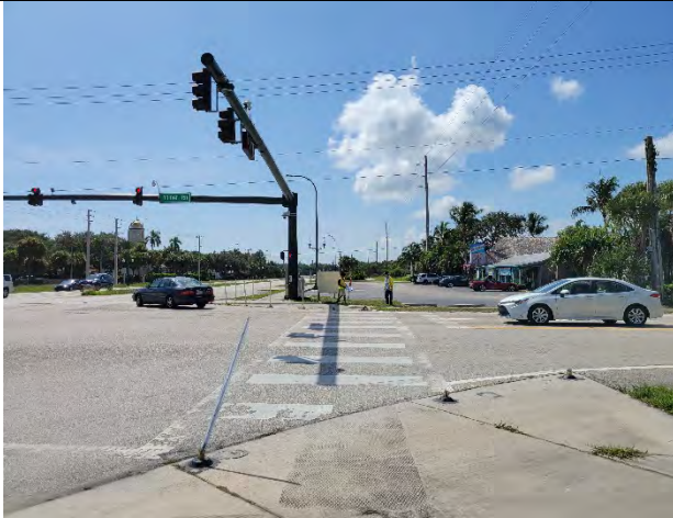
West Leg Crosswalk (NWC) – Multiple Missing Delineators, Missing Tactile Surface
