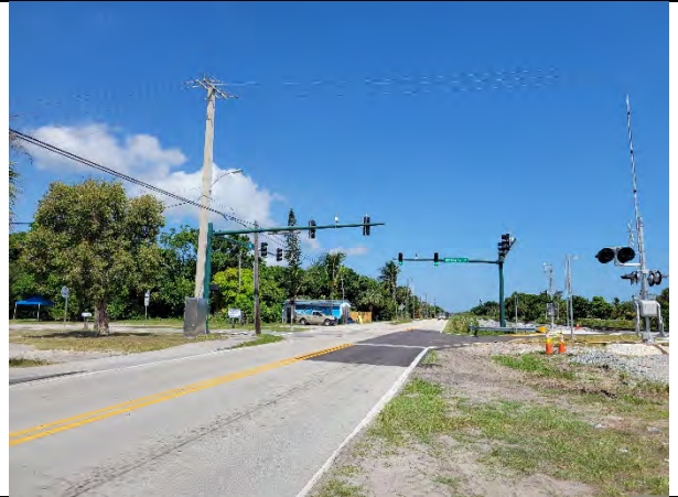
Pettway Street Intersection – Missing Sidewalks East Side – Sidewalk (76") on West Side
