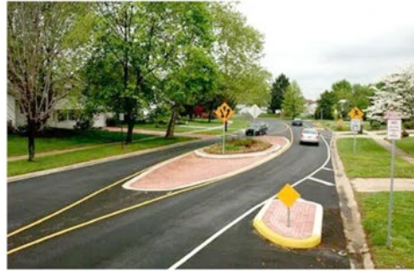
Center Median Island / Chicane
