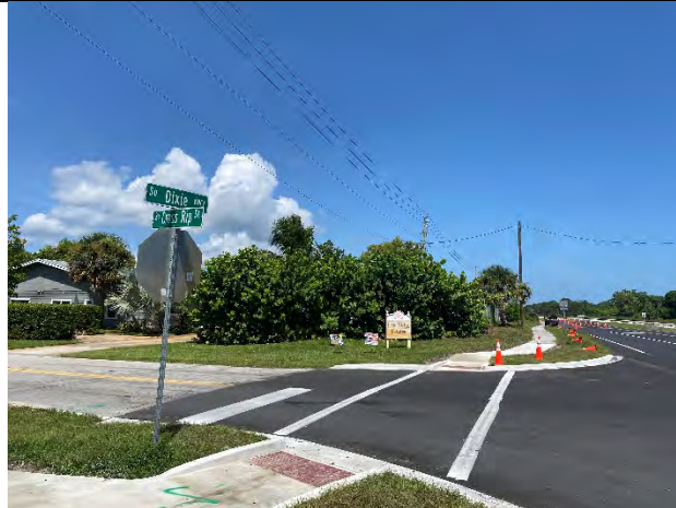
Crosswalk at Dixie Highway and Crossrip Street – West Leg - North
