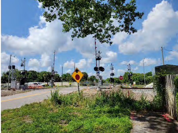
Sidewalks Missing Over Crossrip – West
