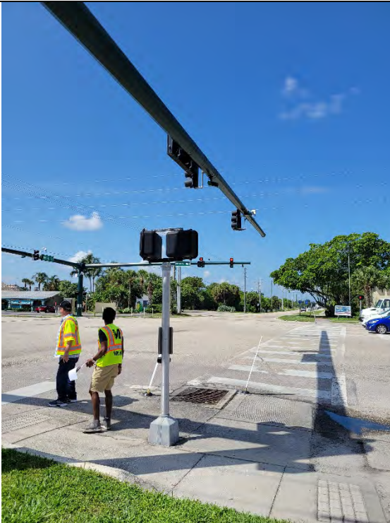
East Leg Crosswalk (NEC) – Missing Delineators and Tactile Surface - South
