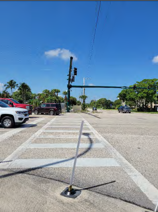
North Leg Crosswalk (NEC) – Drainage Grate, Faded Crosswalks, Delineators Partially Obstructing Pathway, Missing Tactile Surface - West
