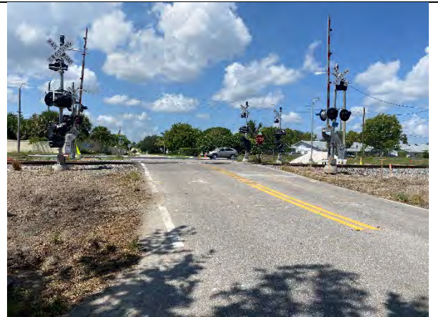
Crossrip Street near Dixie Highway – Sidewalks Missing both sides - West
