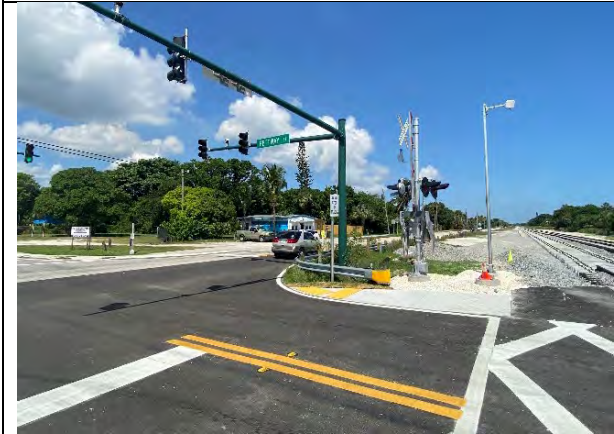
Crosswalks Missing at Intersection of Pettway St - Northwest
