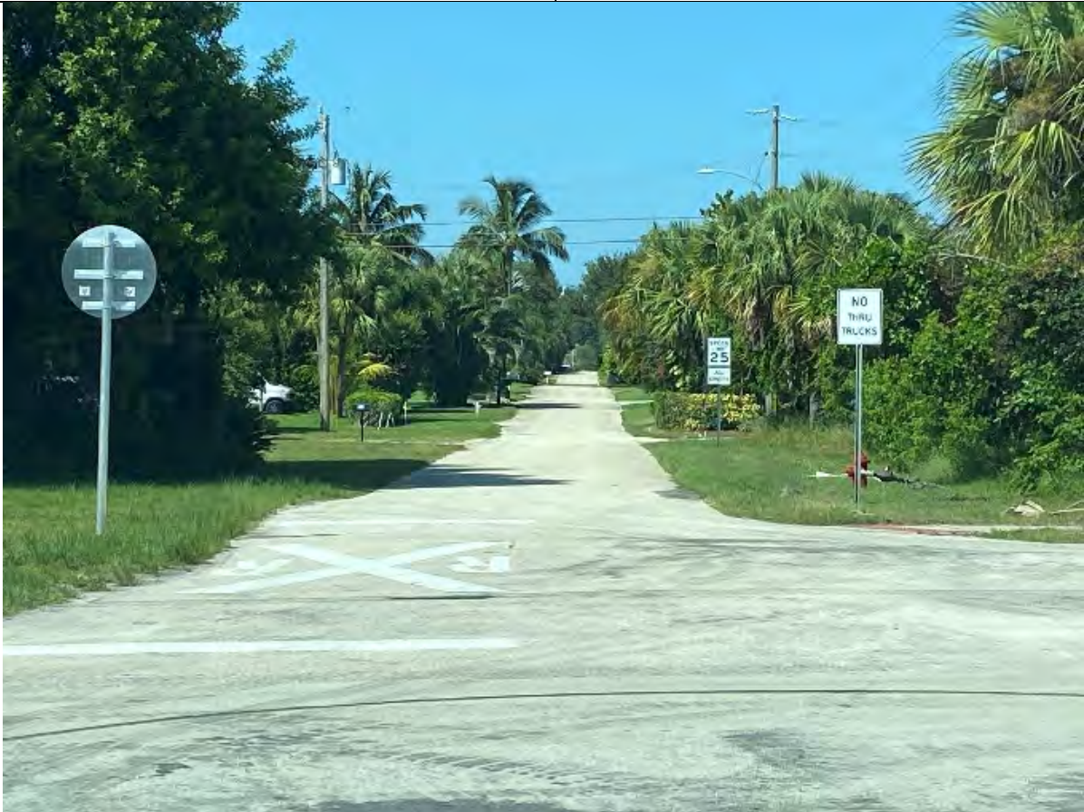
Sidewalks Missing on Gleason/Saturn Ave West of Dixie Hwy
