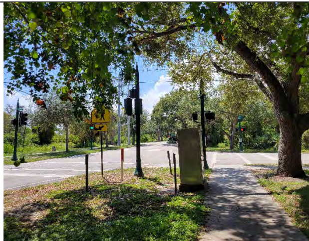
Bridge Road East of Gomez Avenue Crossing and Utilities - West
