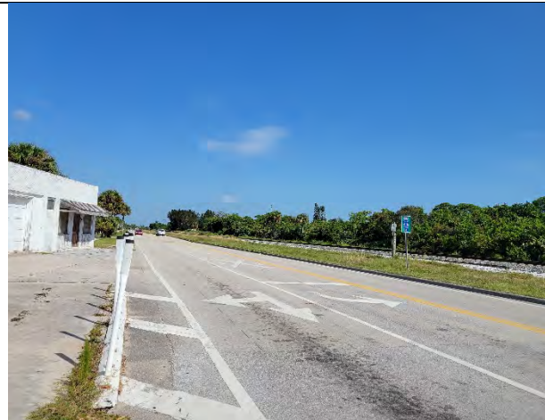
Sidewalks Missing near Bridge Rd intersection - North
