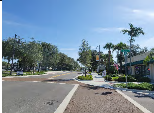
Patterned Crosswalks, Street Lighting - Hercules & Bridge Intersection (SWC) - East
