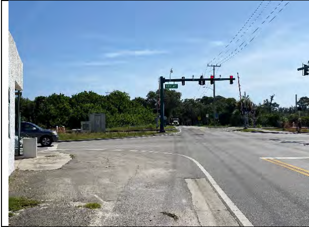
Missing Sidewalks on North Side of Bridge Road at Dixie Hwy Intersection – East
