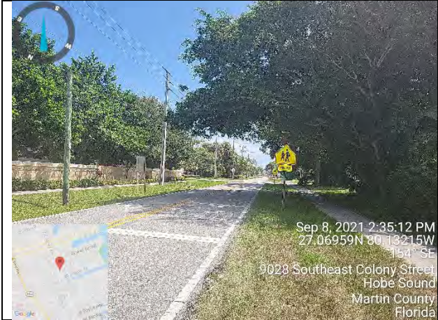
Existing Sidewalks, Utilities in ROW East Side - South
