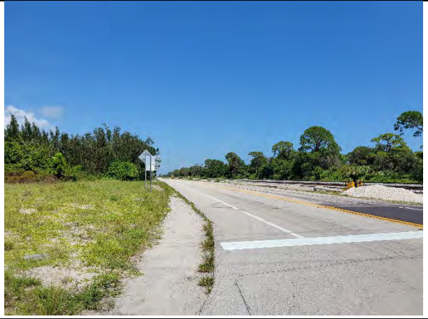
Sidewalks Missing on Both Sides of Dixie Highway, Bike Lanes Present - North of Osprey Street
