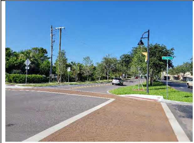
North Side Missing Sidewalk (NEC) – Hercules & Bridge Intersection - West
