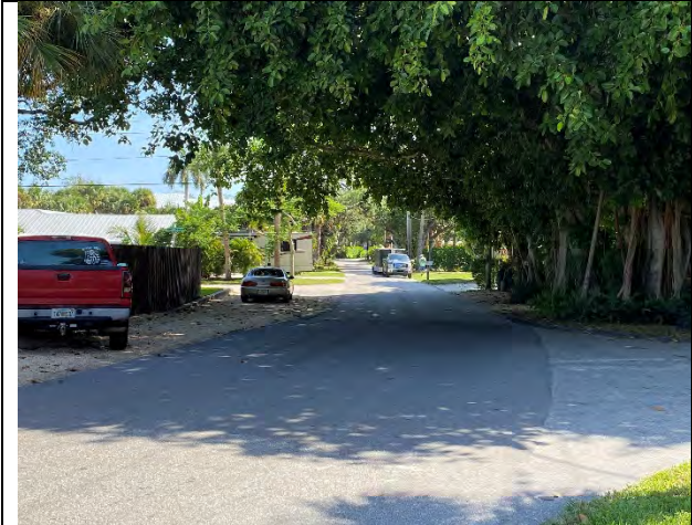
Sidewalks Missing on Both Sides of Gleason Street - East
