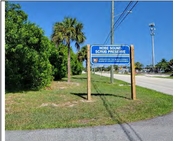
Hobe Sound Scrub Preserve Missing Sidewalks West Side - North
