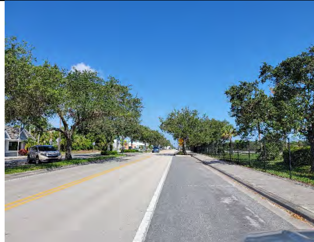
Partial Sidewalk East Side 79", One-Way Perimeter Road on West Side – North
