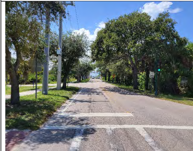
Sidewalks Missing North Side of Bridge Road - West
