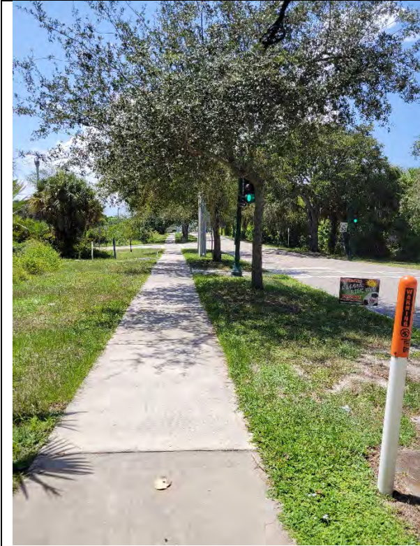
South Side Sidewalk on Bridge Road near Gomez Ave - West
