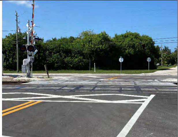
Sidewalks Missing at Railroad Crossing at Gleason and Dixie - West
