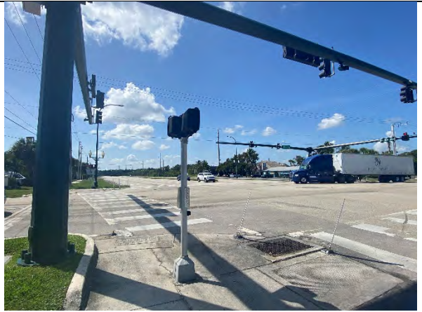
NEC Ped Signal Obstructing Walkway, Drainage, No Curbing, No Tactile Mats - South
