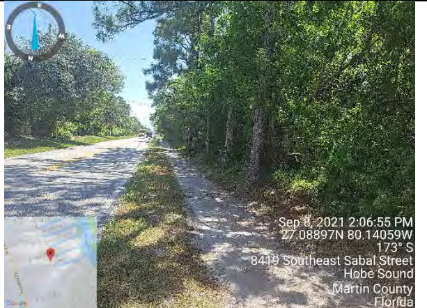
Tight ROW on West Side of Gomez Ave - South
