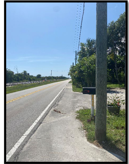
Figure 27: Photo of Significant Pinch point for the Sidewalk along Dixie Hwy (Southbound)
