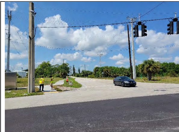
Intersection of Osprey Street and Dixie Highway – Crosswalks Missing, No Ped Signals - West
