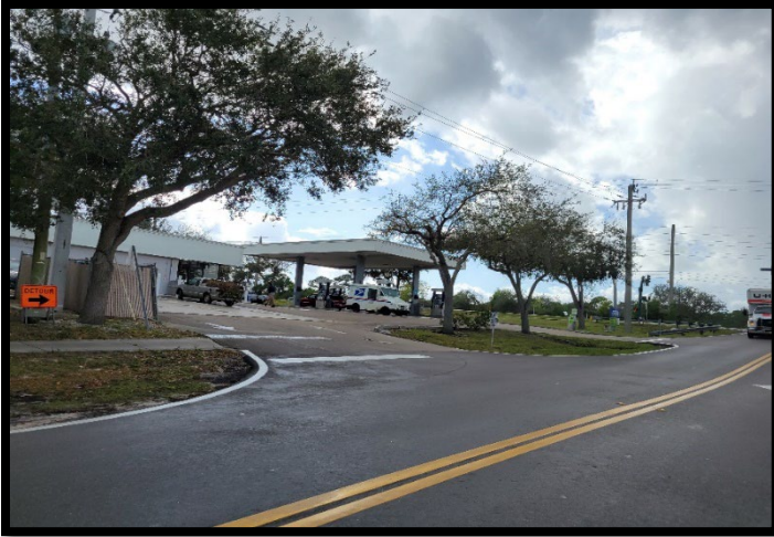
Figure 37: Sidewalk ends at gas station, does not connect to SR-5
