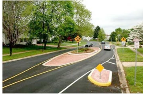
Center Median Island / Chicane
