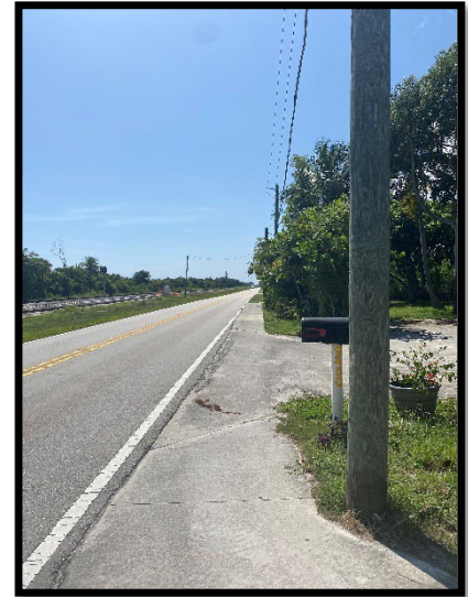
Figure 27: Photo of Significant Pinch point for the Sidewalk along Dixie Hwy (Southbound)
