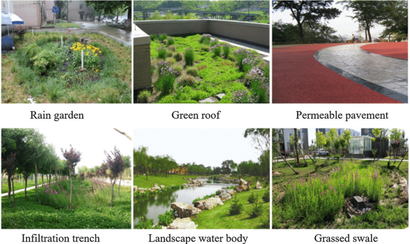
Figure 69: Examples of Green Infrastructure
