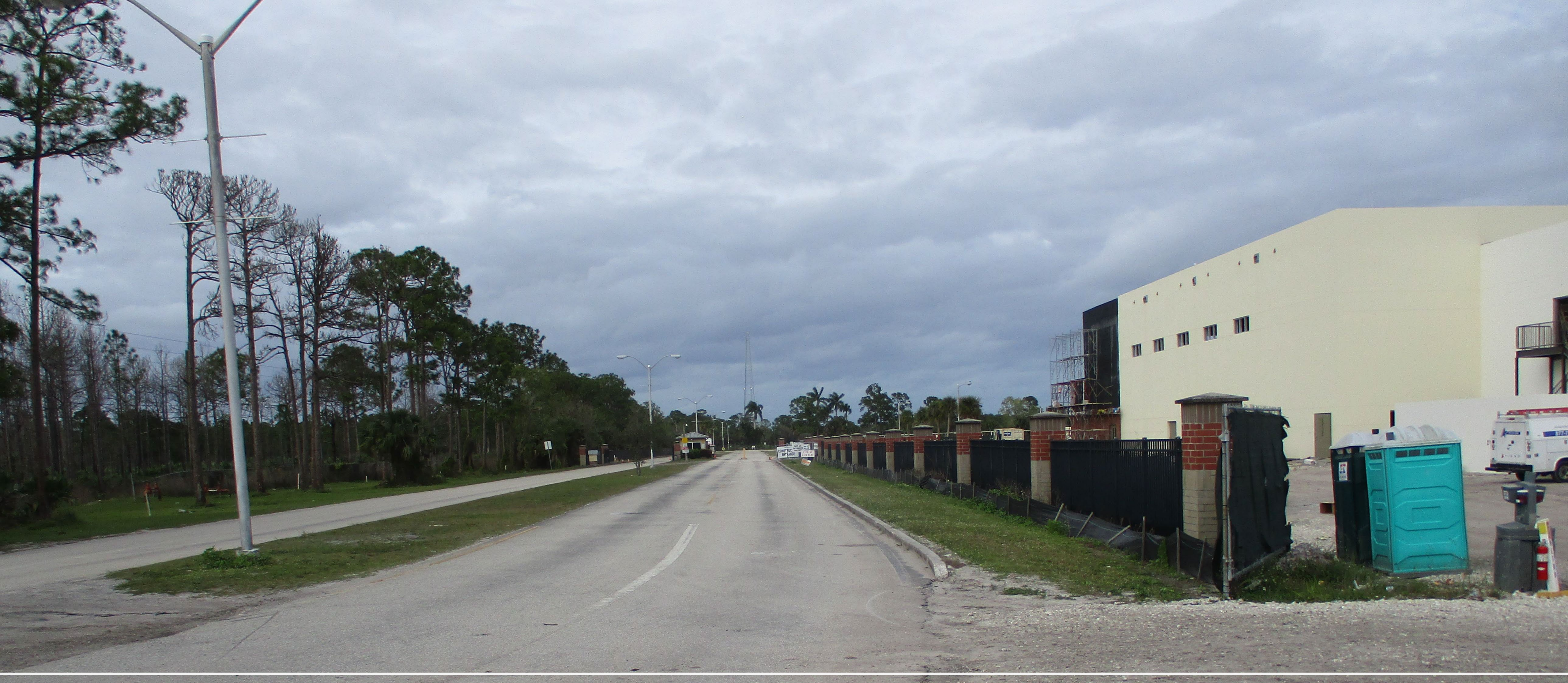
Existing Conditions – SW Bulldog Way at SFHS entrance
