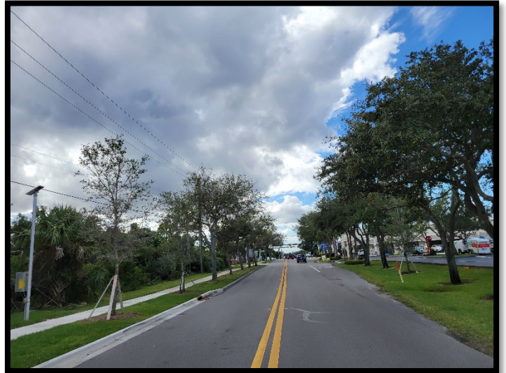
Figure 33: Bridge Rd, looking west
