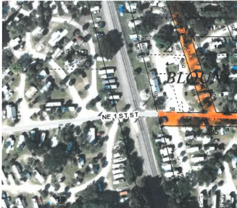
Top Aerial: NE 1 st St / FEC RR Crossing
