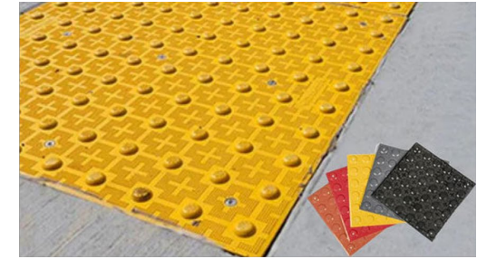
Detectable warning surface example – S03, S06, S08-S10
