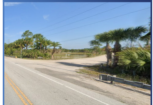
SW Springhaven Avenue Design Underway, Construction Planned for 2027
